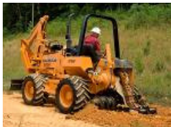
The Astec RT960 trencher at work
