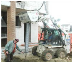
The U.Emme self-loading mini batcher/mixer makes light work of pouring pilings and footings
